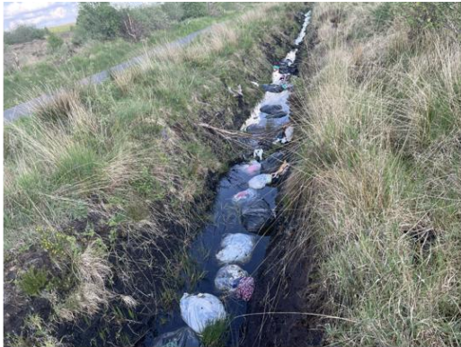
View of roadside drain at the target note 5 location. The drain is on south side of public road separating the study area from the Cloonashanville Bog SAC to the north. Note fly tipping in drain
