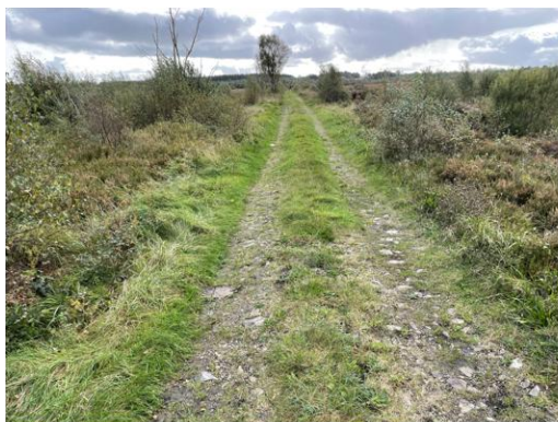
View of target note 42 existing access road leading to T03 location. Road has since been resurfaced
